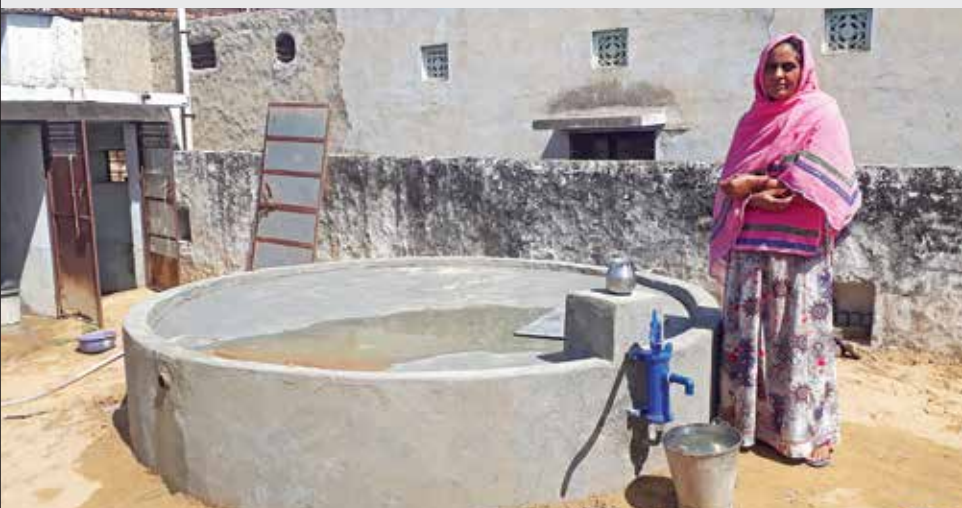
Roof Rain Water Harvesting Structures (RRWHS) has proved a one time investment and permanent solution to pure and safe drinking water. Suman Kanwar of village Kasli with her RRWHS structures in Sikar.
