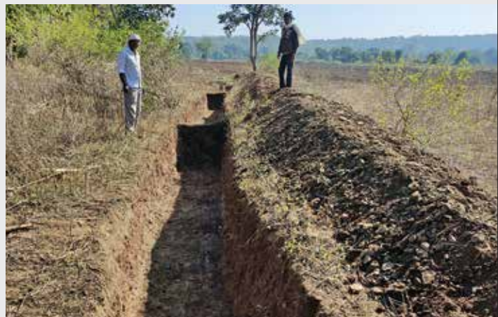
WAT (Water Absorption Trench) is a trench which absorbs water and reduce the soil erosion. A WAT constructed in the field of farmer in village Nandora Karanja block of Wardha.
